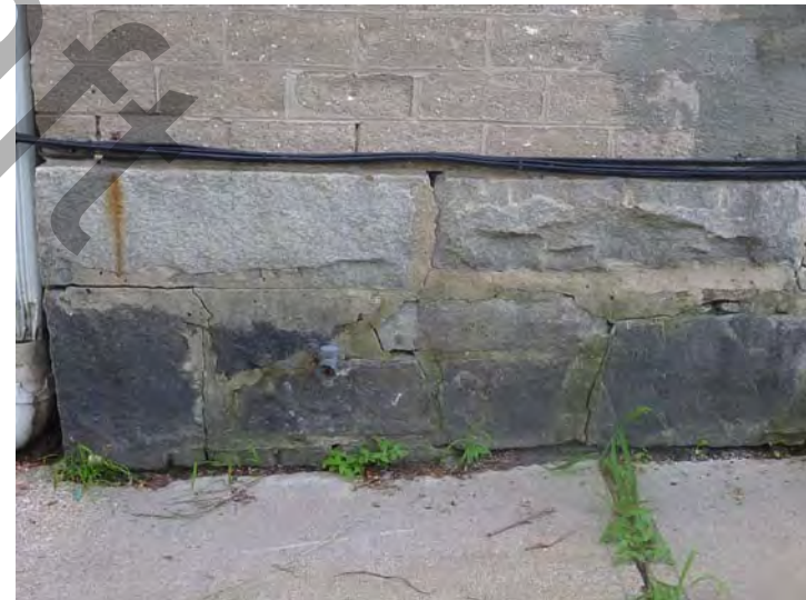
Stone foundation wall crack repair at Building 119 is shown in Year 1 and periodically over the plan.
