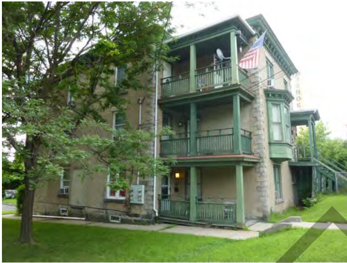
Replacement and painting of wood stairs, decks and rails is shown in Year 1.
