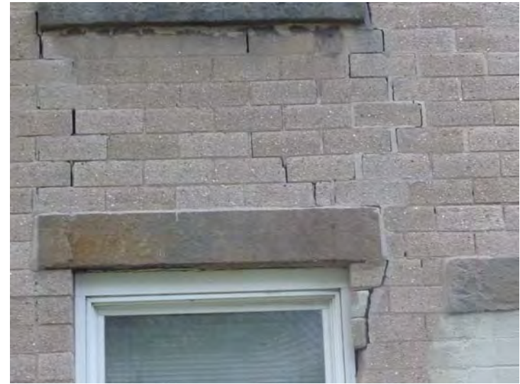
Brick and stone crack repair at Building 119 is shown in Year 1 and periodically over the plan.
