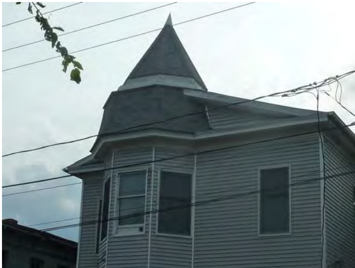
Visible roofing at Building 115 appears in good condition. Roofing at cupola is shown to be replaced early in the plan based on EUL and condition.
