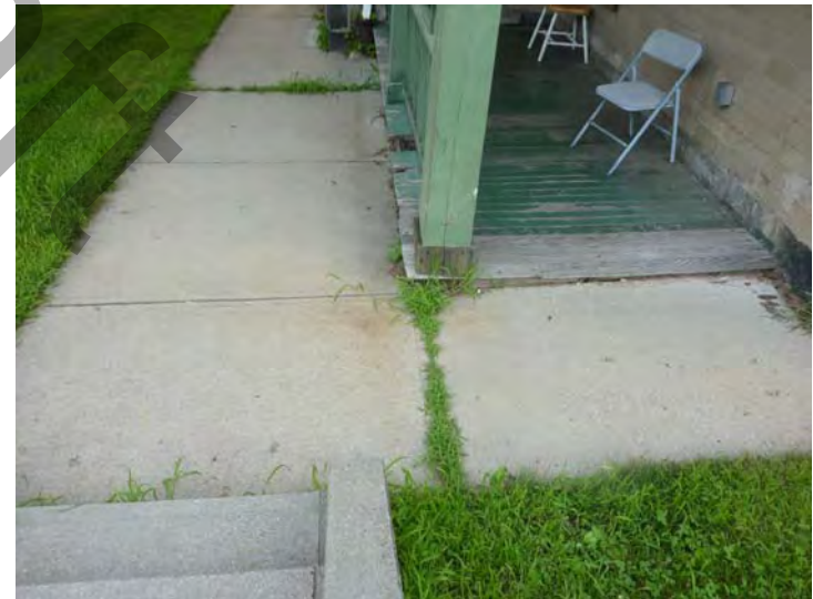
Trip hazards at concrete pavement joints and concrete pavement misaligned with wood deck are shown to be eliminated in Year 1.
