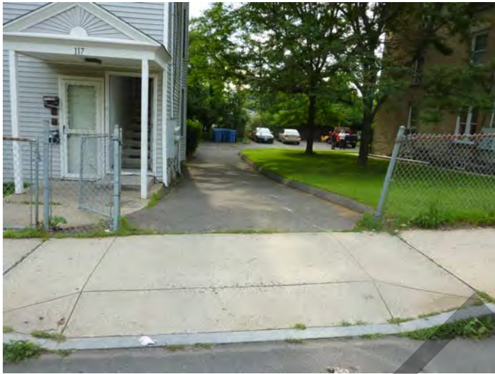
Asphalt paving at drive and parking lots is shown to be crack filled and seal coated periodically over the plan.
